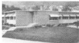
Creston substation, constructed in 1957.
